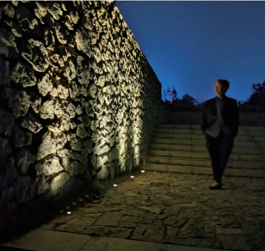
Pathway or gate post where anti-glare luminaires are required.
