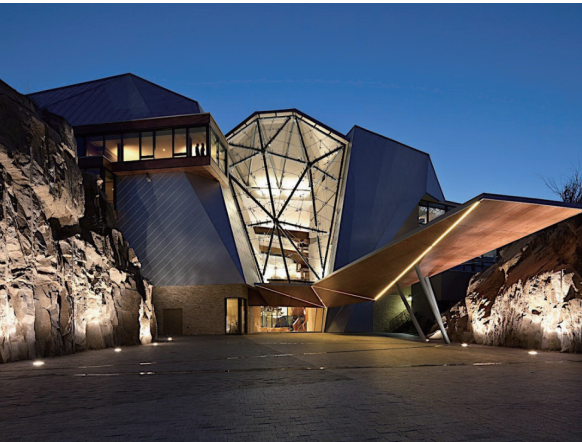
Plaza illumination where the anti-glare is necessary
